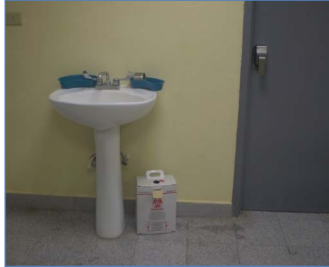
Before: Sharps box insecurely stored
